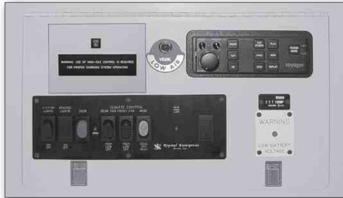
F-550 Overhead Control Panel
