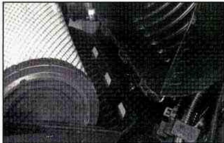
Install the new filter by pushing it all the way to the stop on the duct.
